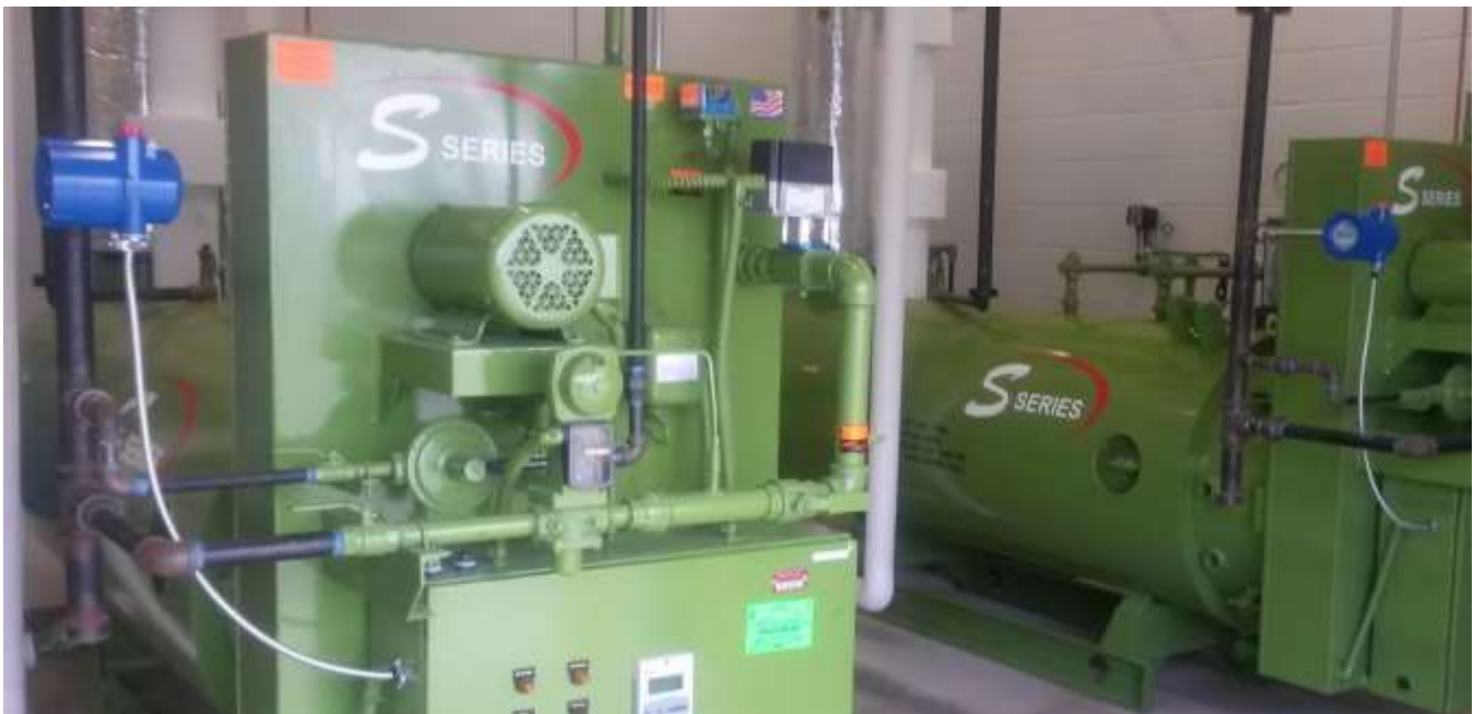
Figure 6: Two Thermal Mass Gas Flowmeters measuring natural gas flows on 2-boilers at a manufacturing facility.
