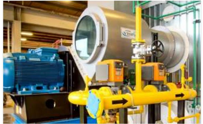
Figure 3: *The VISION Burner technology ensures complete and efficient combustion with very low emissions; < 30 ppm NOx with low FGR rates.*
