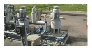
Liquid waste from compressor station scrubbers & filters can be condensates or hydrocarbons from the natural gas. The wastes are collected in one or several tanks depending on the size of the remote station. Waste tank trucks are scheduled for emptying operations that are classified as hazardous materials. **Challenges:** These condensed hydrocarbons and condensed water tanks can overflow or run pumps dry when the level becomes too low.
