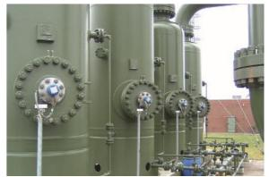
A typical compressor station consists of an inlet scrubber to collect liquids and slugs that may have formed in the gas pipeline. The scrubber consists of a primary section where liquids and solid parts are separated from the gas stream and a secondary section where the oil mist is removed from the pipeline.
