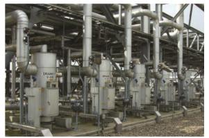
A Vapor Recovery Unit (VRU) captures valuable VOC's and other rich gas streams that may be a significant environmental pollutant. A VRU collects from storage and loading facilities, re-
