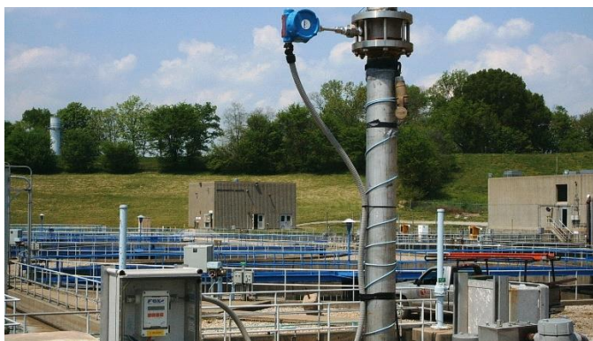
Figure 2: Fox FT2 air flowmeter on an application for a waste treatment plant in 2005.
