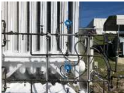
Figure 1: Thermal mass flow meters excel in N 2 flow measurement for bulk tank farms, Argon for welding gas lines, CO 2 for bottling process, He for GC's, H 2 for Gen Sets and Methane for fuel.
